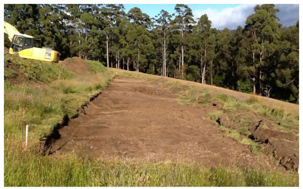
Plate 1 (above). This NCB was sized to Category 6 on-site subsoil, but with 0.3 - 0.4m of Category 4 topsoil. Accordingly, it could be constructed as a cut-and-fill operation where the outer edge is built up using soil from the inner edge.
