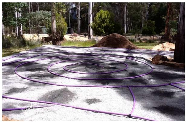
Plate 5 (above). The pump pit is filled with water, a few initial 3 - 4mm diameter holes drilled at random in the pipework, and the pump turned on. Add more drill holes, nominally at about one metre centres, as the outflow from each is checked to ensure even coverage.
