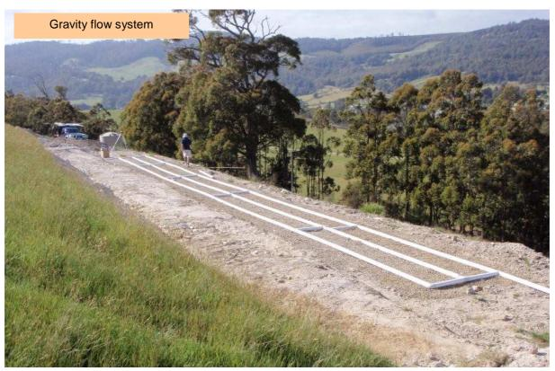
Above. This nonconventional bed received gravity flow wastewater from a septic tank up the slope at right.
