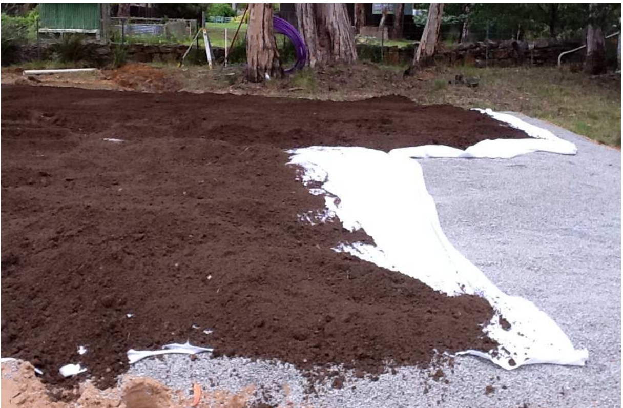
Plate 6 (below). Cover pipework with aggregate, filter cloth and nominally 150mm of loam before landscaping.
