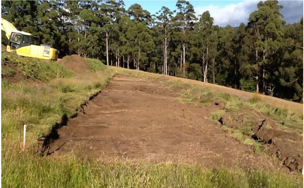
Plate 1 (above). This NCB was sized to Category 6 on-site subsoil, but with 0.3 – 0.4m of Category 4 topsoil. Accordingly, it could be constructed as a cut-and-fill operation where the outer edge is built up using soil from the inner edge.
