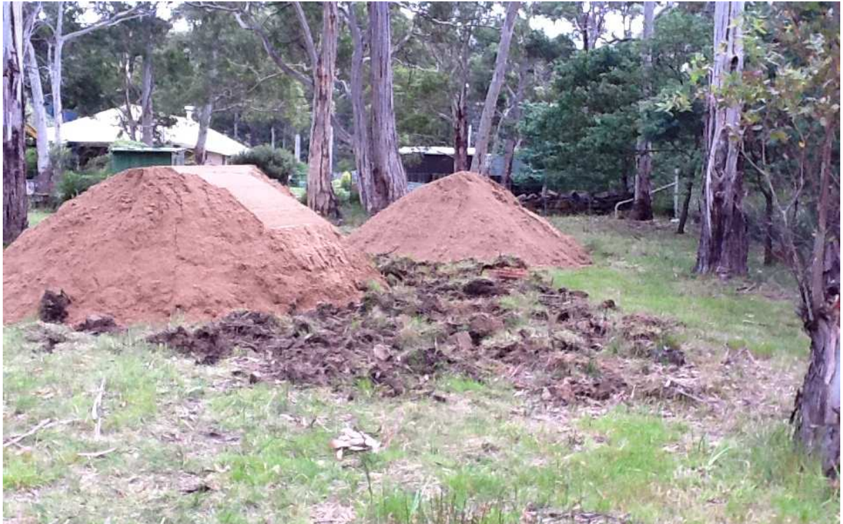
Plate 1 (above). Rip beneath basic module; stockpile filter sand. The soil is Category 6 clay to the surface. The PDA is sized to account for this, using a DLR of 3mm/day.
