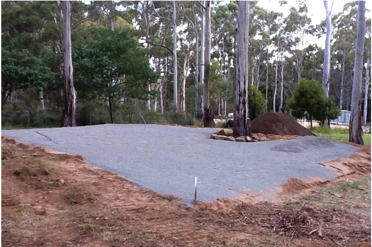
Plate 3 (above). Place and level nominal thickness of 50mm of durable, clean screened aggregate over the filter sand.
