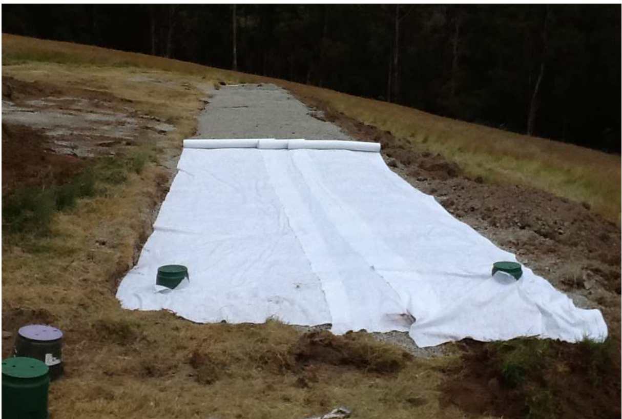
Plate 8 (below). Filter cloth cover over aggregate
