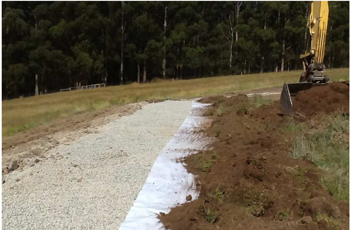
Plate 9 (above). Final cover of 150mm loam before landscaping.
