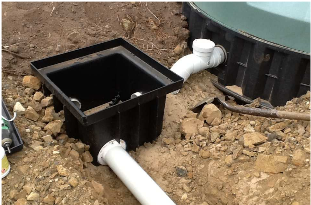
Plate 10 (below). A two-way distribution box after the septic tank directs wastewater equally to each of two equally-sized PDAs.
