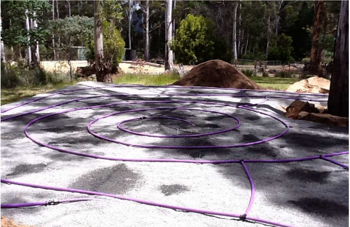
Plate 5 (above). The pump pit is filled with water, a few initial 3 – 4mm diameter holes drilled at random in the pipework, and the pump turned on. Add more drill holes, nominally at about one metre centres, as the outflow from each is checked to ensure even coverage.
