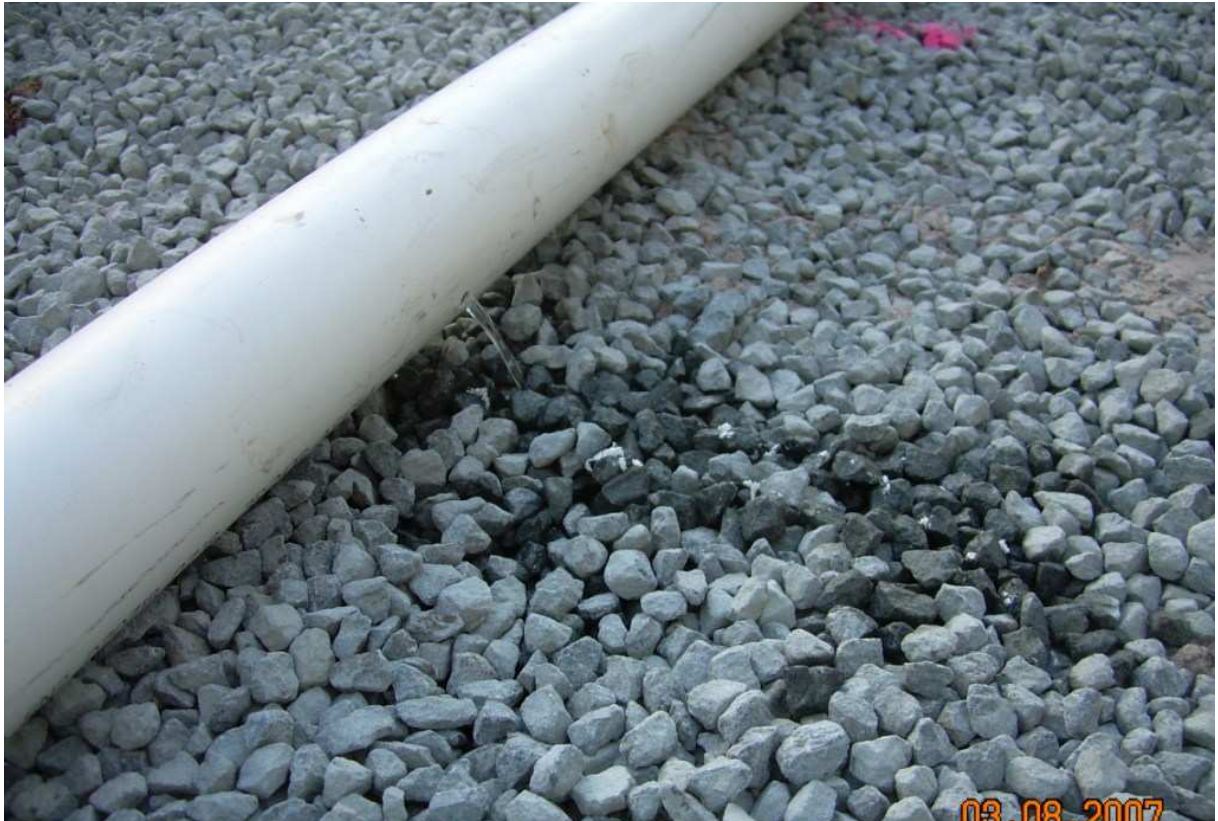
Plate 5 (above). Perforated pipework under test. Photo: Bill Cromer
