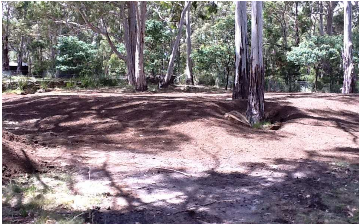
Plate 2 (below). Spread and level filter sand to required thickness; batter the sides.
