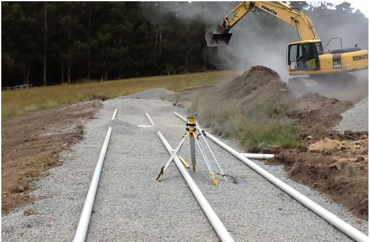
Plate 6 (below). Pipework perforated, levelled, tested and being covered with aggregate.
