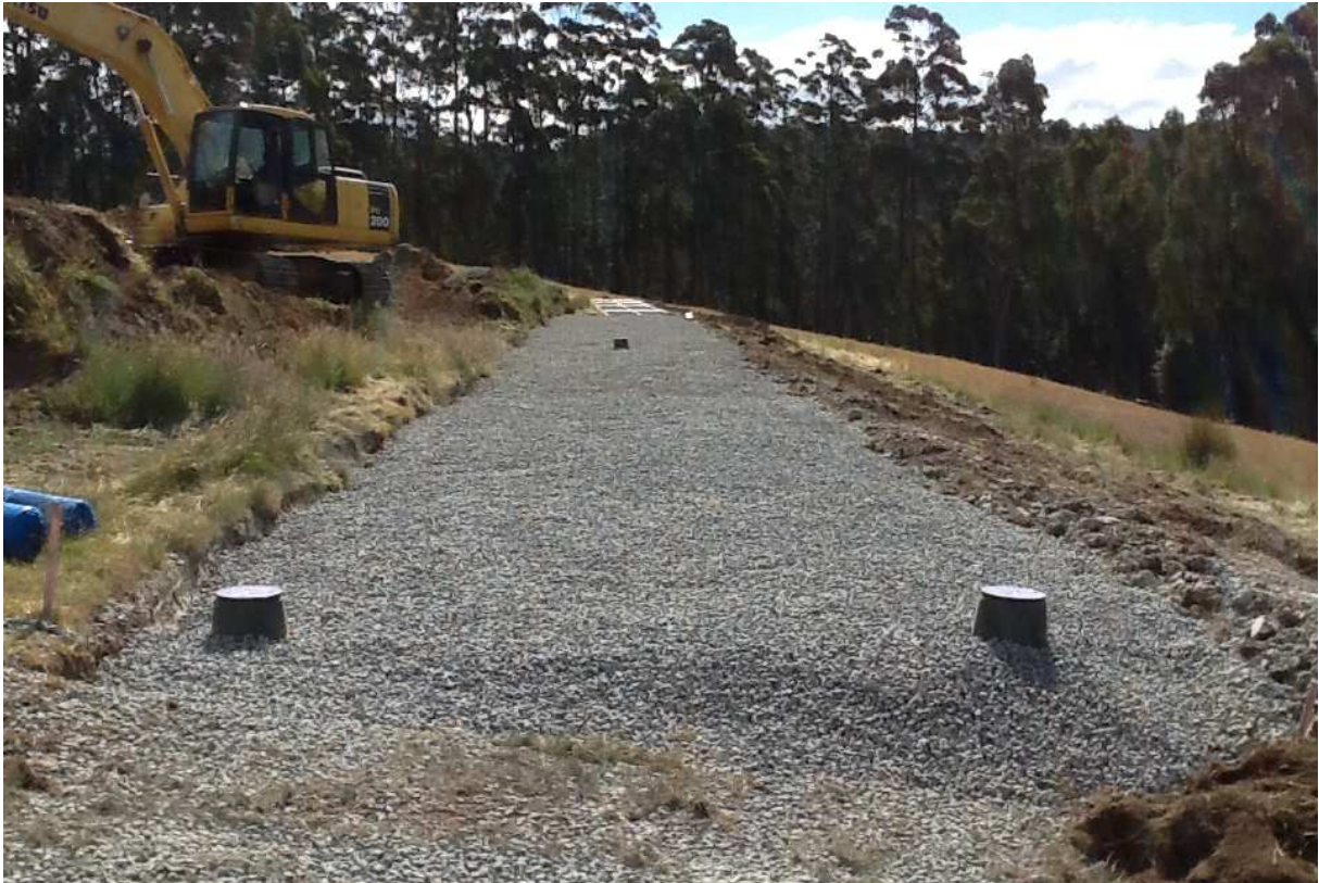
Plate 7 (above). Screened aggregate covering distribution pipework. Inspection openings extended to final surface
