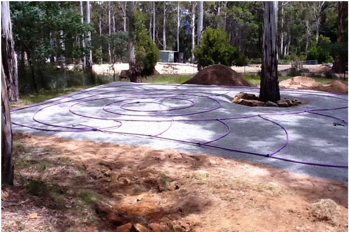
Plate 4 (below). Lay unperforated, colour-coded 25mm polyethylene pipe over the aggregate.
