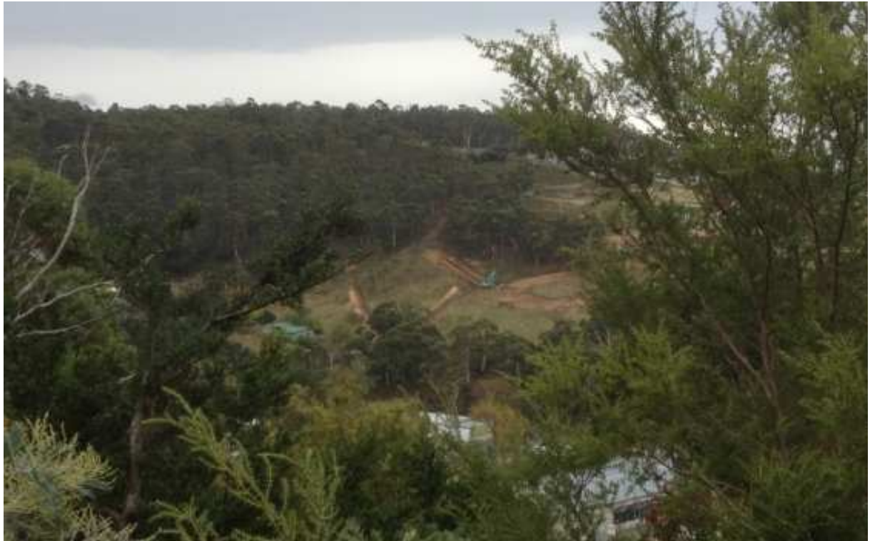
Plate 1 (above). View north from Wellerslie Park in South Hobart to Lot 47 on the Farm Hill Subdivision in April 2014, showing service trenches (right) and investigation trenches B and D ("V"-shaped).
