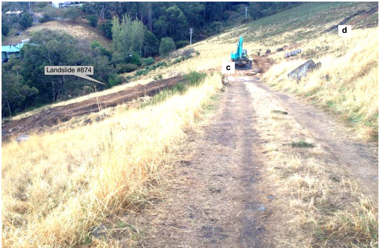
Plate 8 (below). View northwest and downslope in March 2014 towards the service trench a....f. Lot 47 is the grassy slope in the background. The higher edge of the tree line in the left middle ground marks the headscarp of landslide #874 (see Map 1 of Attachment 5).
