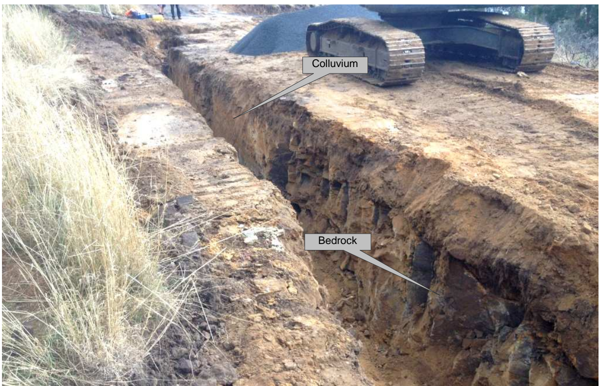
Plate 12 (below). Service trench abcdef at c, but opposite side of trench to that in Plate 11.
