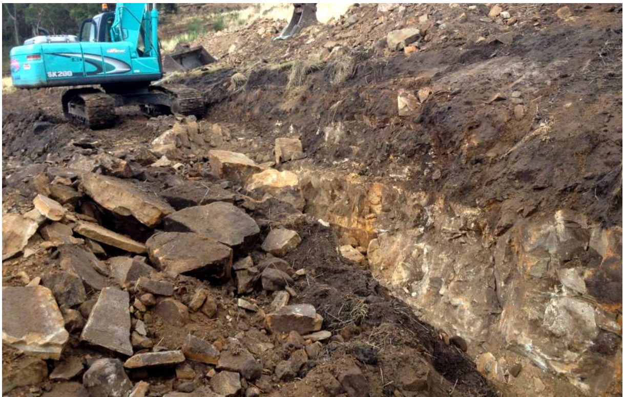
Plate 10 (below). Service trench abcdef between b and c. Subhorizontal Triassic sandstone bedrock exposed at depths less than 1m.
