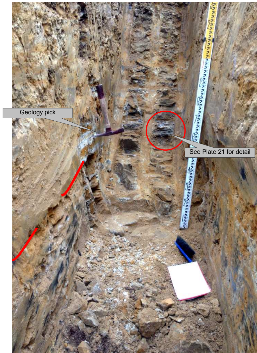
Plate 20 (left). Investigation trench B, upslope end, showing finely bedded, highly weathered sandstone and siltstone bedrock dipping 3^{\circ} to 017^{\circ} T. Colluvium (with some bedded sandstone) overlies the bedrock, and the boundary (red line) between them, although not very obvious, is inferred to dip towards and up to the camera in a scallop shape (the geology pick is on the boundary).
