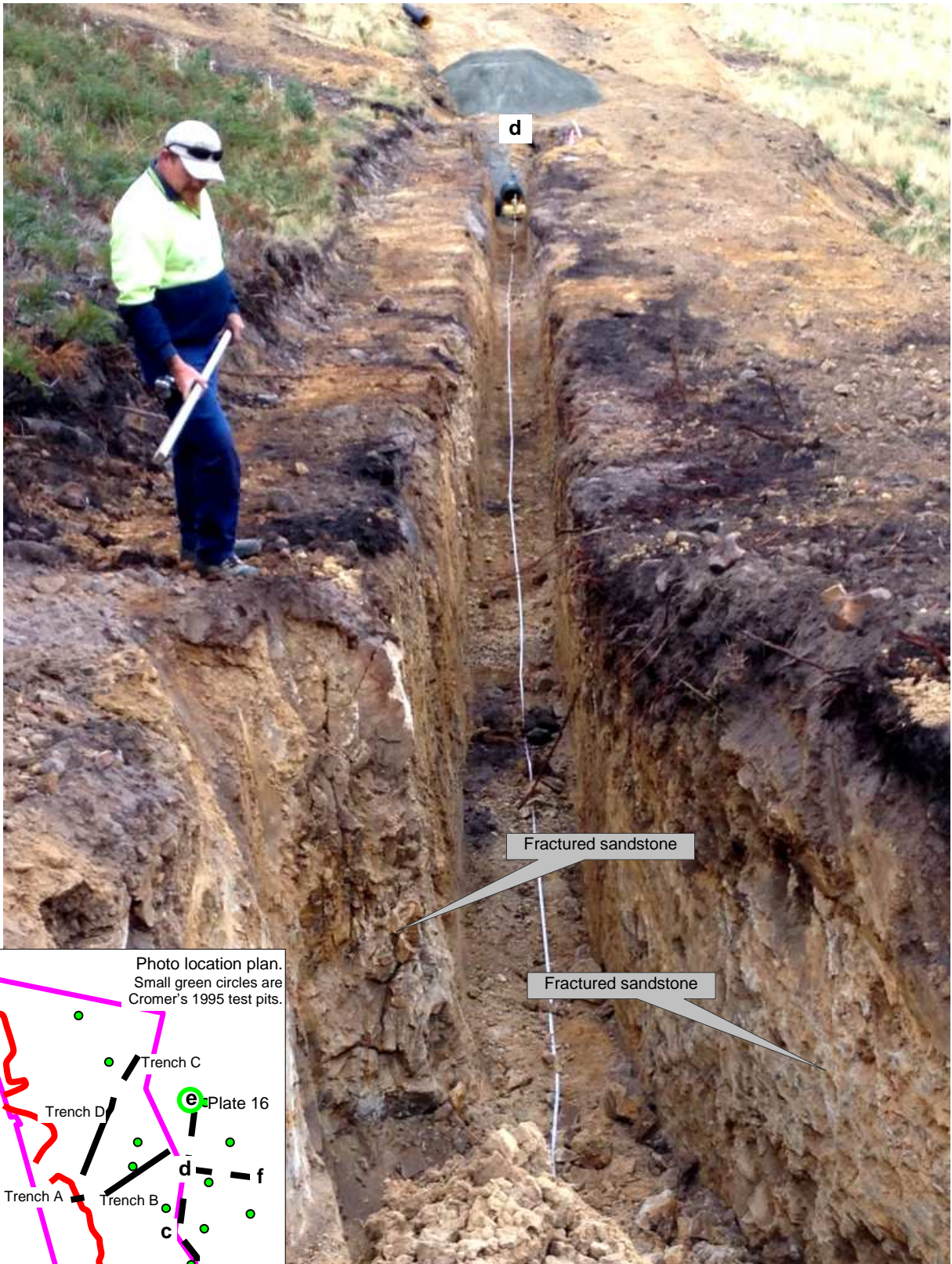
Plate 16. Service trench abcdef at e, looking downslope to d. It is not clear whether the fractured sandstone exposed in the services trench at this location (and locally elsewhere along it) is in-situ or not.
