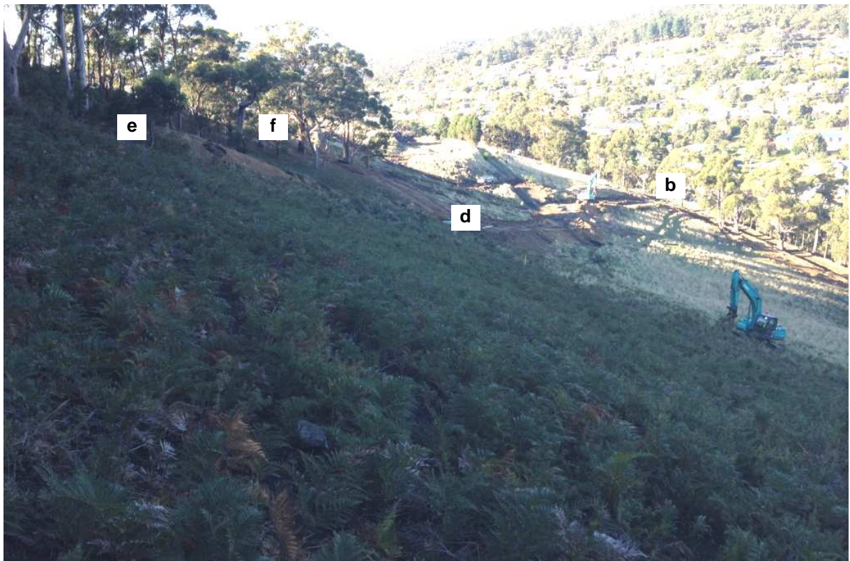
Plate 2 (below). View southeast from the northwestern corner of Lot 47 at Farm Hill, over 25 – 30° slopes in the foreground, towards service trenches a....f (see Attachment 7).
