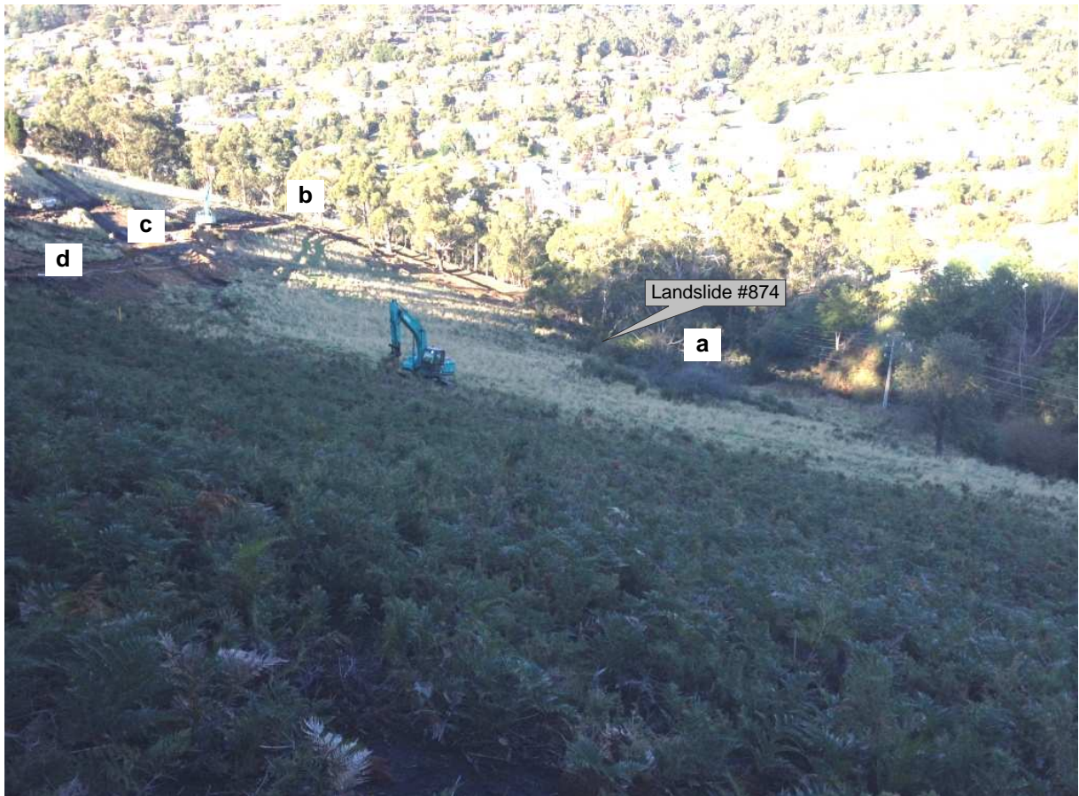
Plate 3 (above). View south southeast from the northwestern corner of Lot 47 at Farm Hill, over 25 – 30° slopes in the foreground, towards service trenches a...f (see Attachment 7). The higher edge of the tree line in the centre of the photo marks the headscarp of landslide #874 (see Map 1 of Attachment 5).
